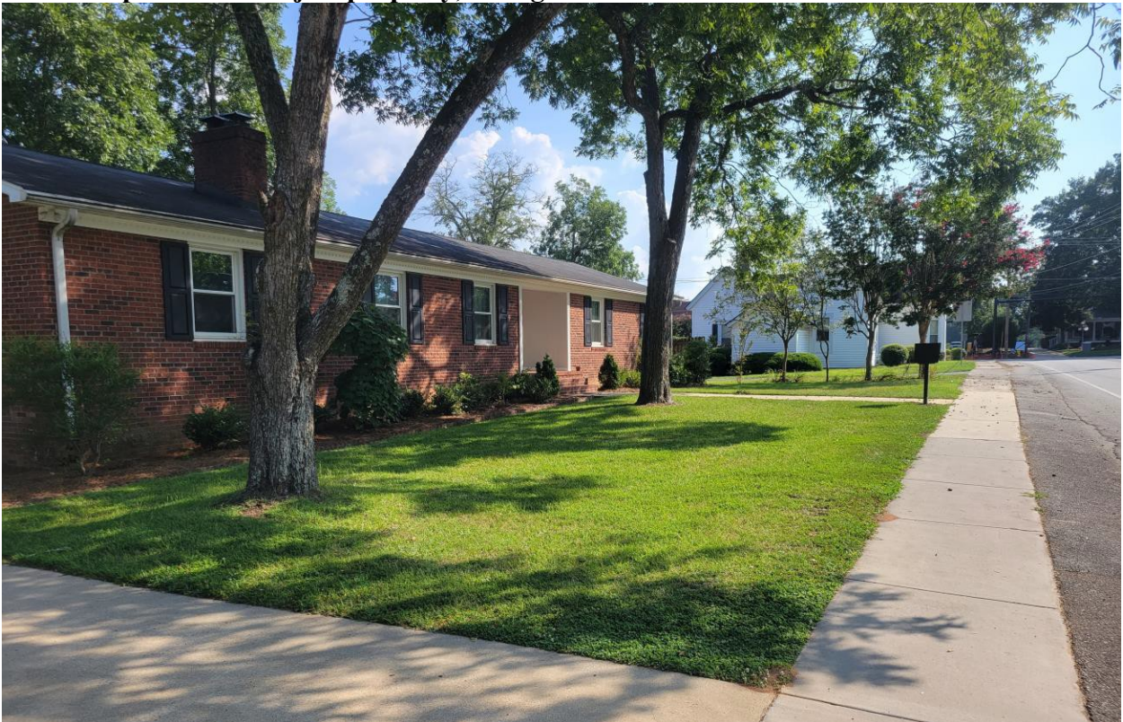
Southern portion of subject property, facing southeast
