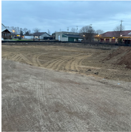
Site Prep - Photo Credit Clarendon Properties
