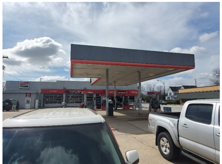
Front of fuel island canopy (no existing sign)
