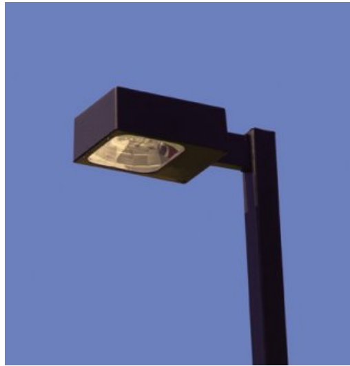
SIMILAR “SHOEBOX” CUT-OFF FIXTURE FOR COMMERCIAL/OFFICE PARKING
