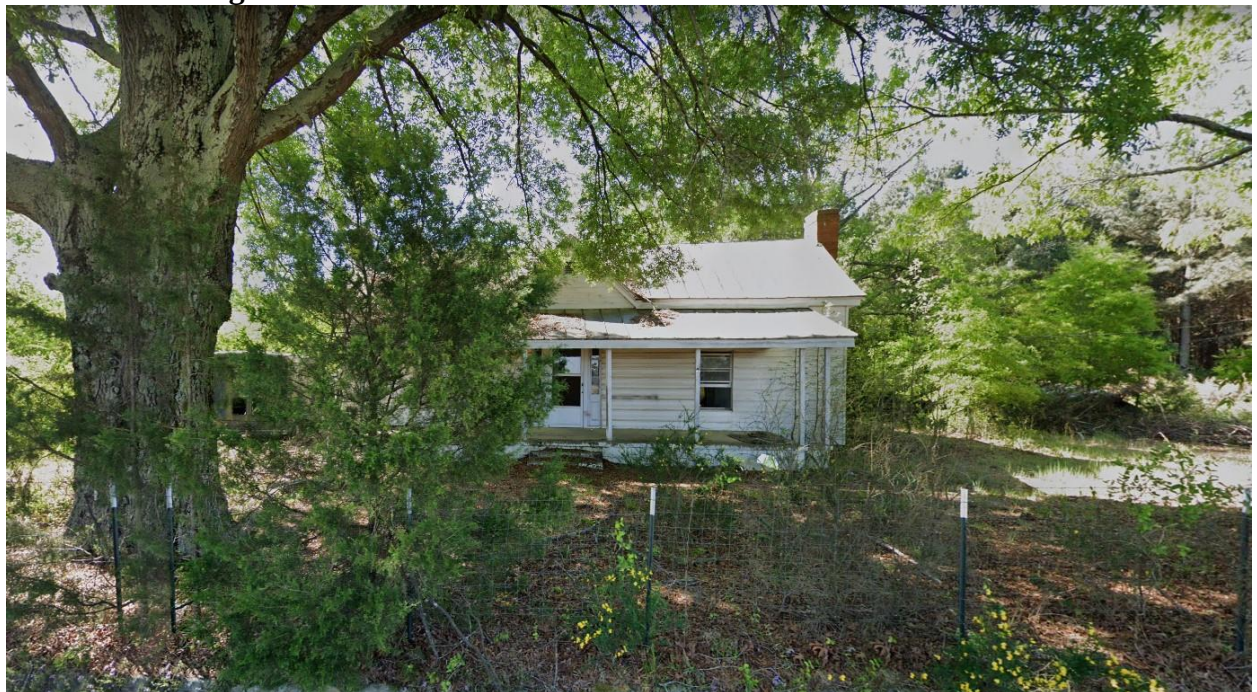
207 Wilson Bridge Road:
