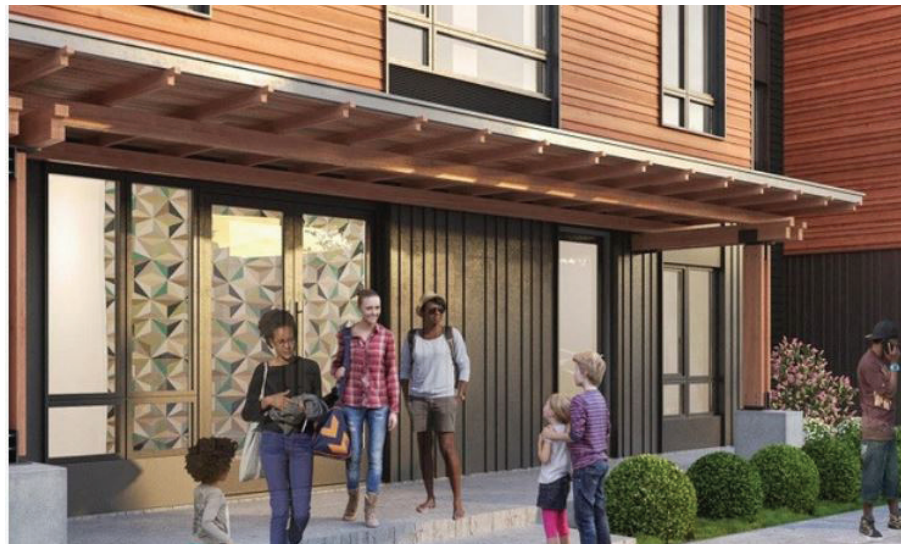
HEAVY TIMBER/ STEEL ENTRY CANOPY
