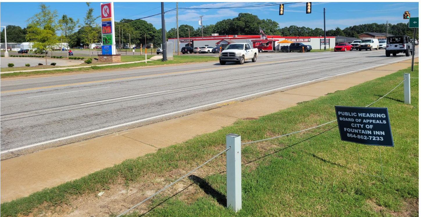
Proximity of enclosed area to the sidewalk, intersection
